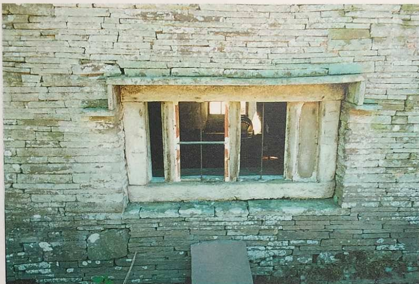
PLATE 3 DIAMOND STUDDED MULLION WINDOW (NORTH ELEVATION)
