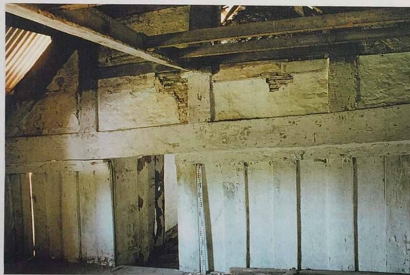
PLATE 6 INTERNAL VIEW OF WESTERN 'A' FRAME WITH CLOSE STUDDING
