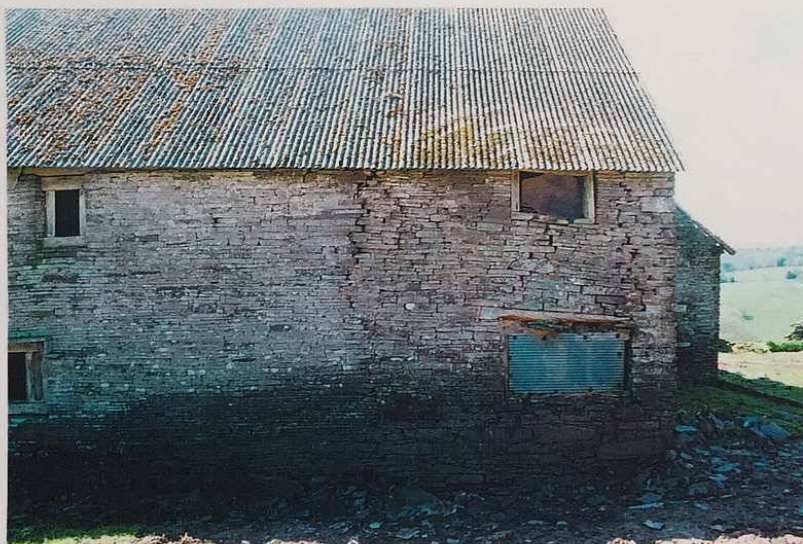
PLATE 4 NORTHERN ELEVATION SHOWING SUBSIDENCE
