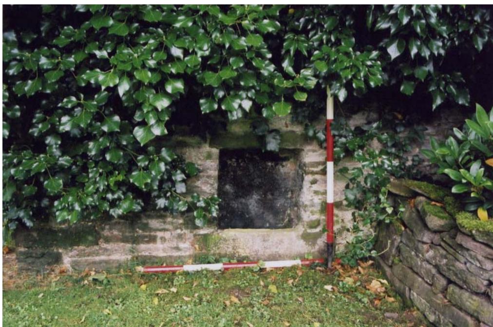
Plate 8: Stone opening for feeding shute, as seen from the garden
