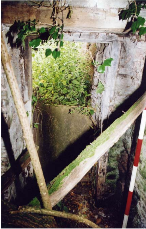
Plate 3: Timber-frame doorway into the old pig pens
