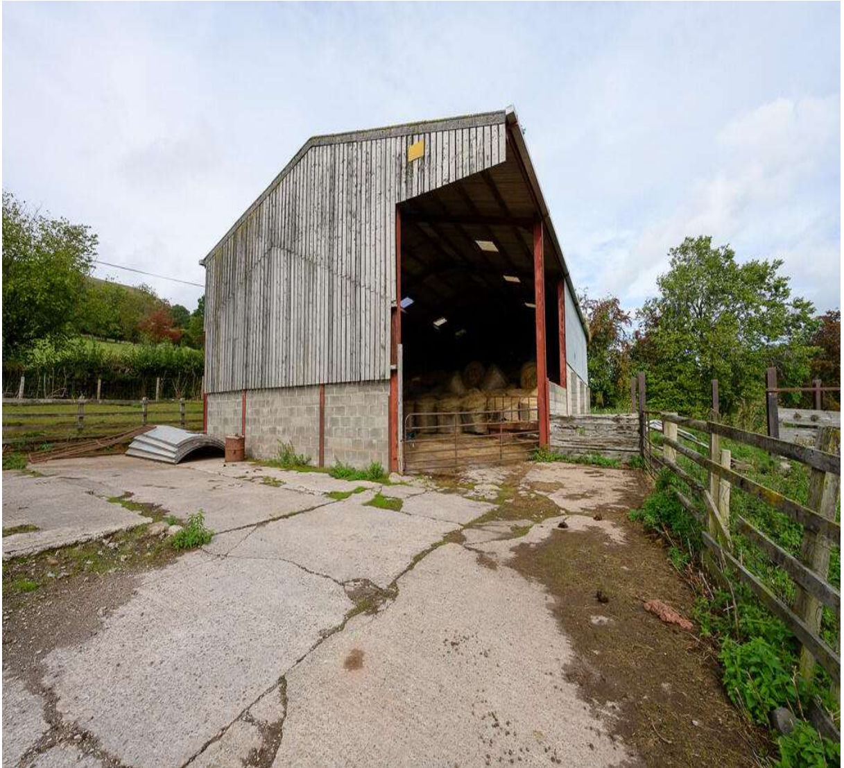
5 of 7Olchon House Farm barn
