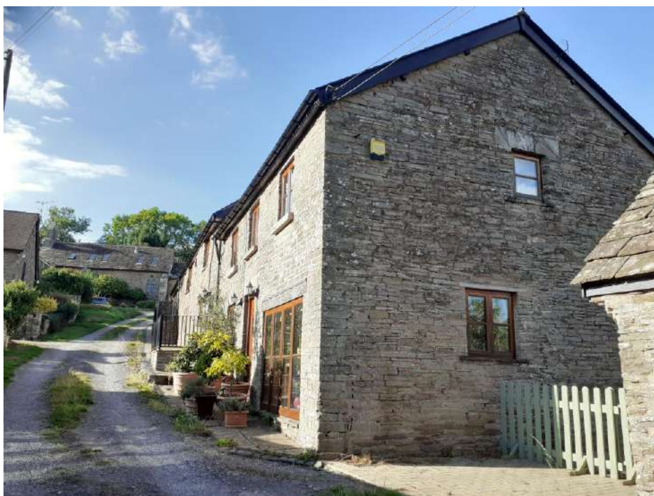
Plate 18: View looking N showing rear elevation of The Ferns, with former church of St Peter's visible in background
