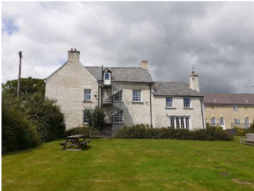
Plate 10: View NW towards the Grade II listed Outdoor Centre (formerly the New Inn) with modern extension visible to rear
