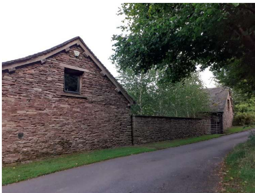
Plate 22: View looking WSW from Mountain Road towards converted outbuildings to S of Lower Turnant
