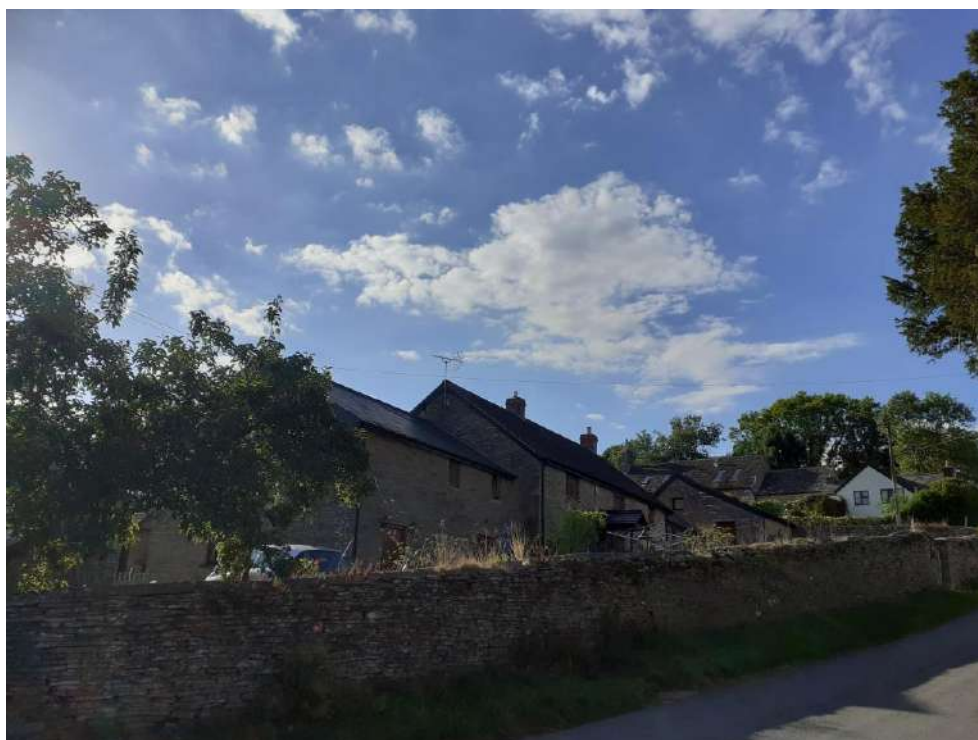
Plate 17: Oblique view looking NW from the main street towards The Ferns
